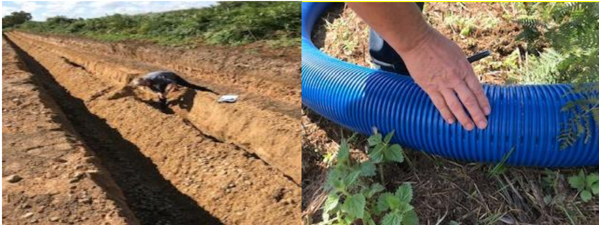
Figure 6. Recharge trench under construction and perforated recharge pipe
